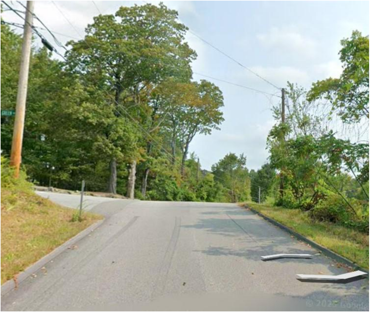
Figure 3. Vertical crest (hump) limiting stopping sight distance at Christian Hill Road and Green Road.
