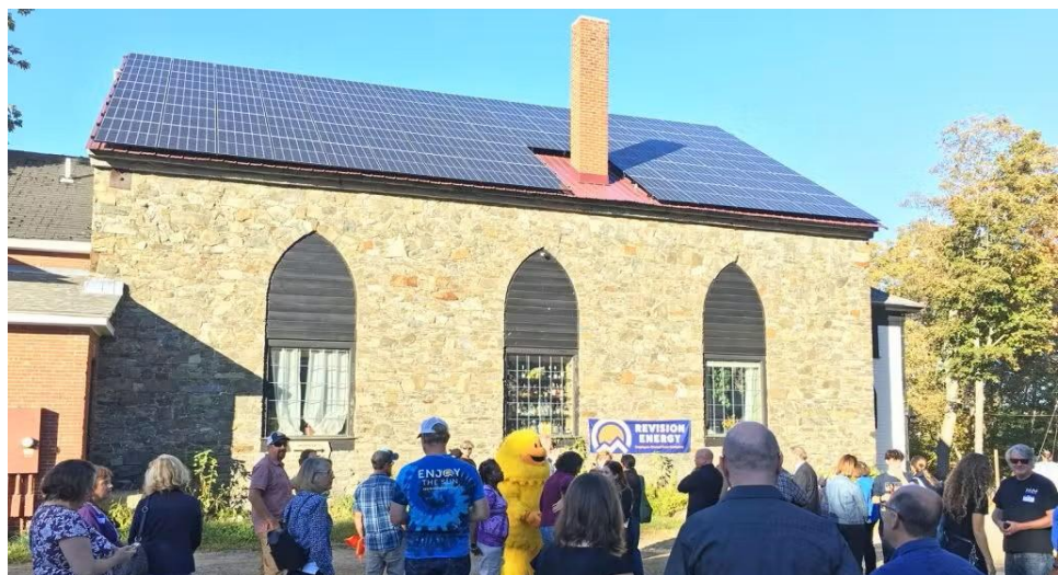
Figure 3 Stone Church Solar Panels (source: Revision Energy)
