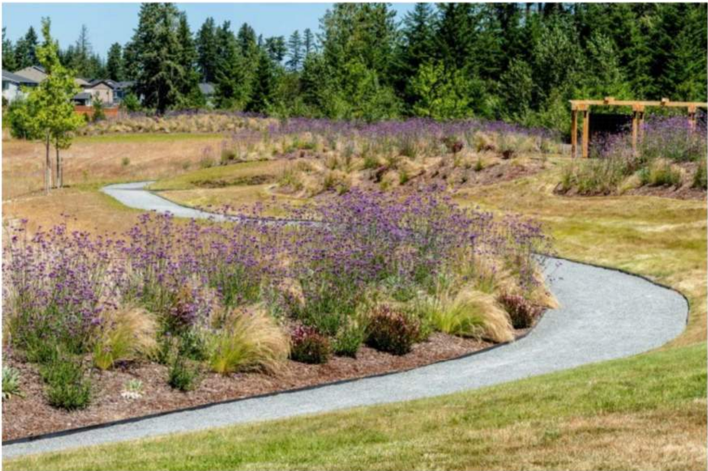
Stablized Stone Dust Path
