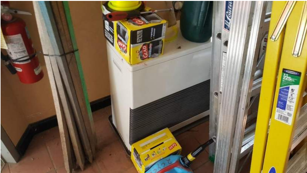
Abandoned Point of Use Fuel Oil Heater
