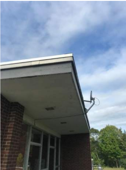
Town of Belmont, New Hampshire Police Facility and Main Street Bank/Post Office Building Existing Conditions Report
