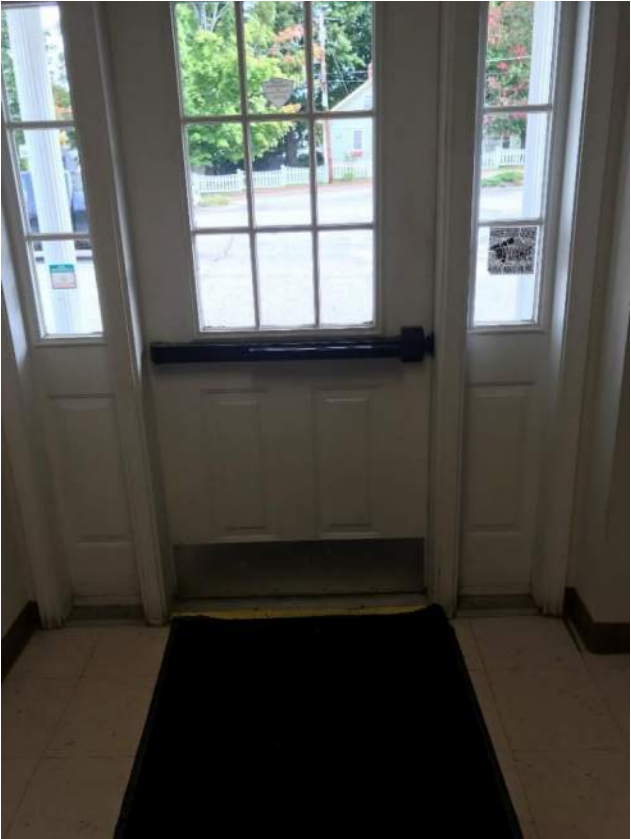
Main Entry – Interior
