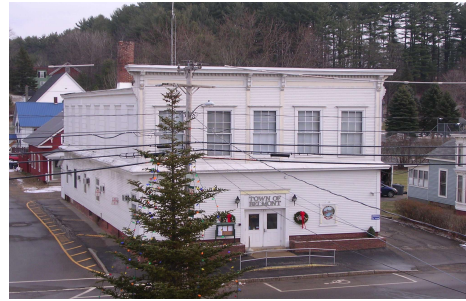
Belmont Town Hall Building
