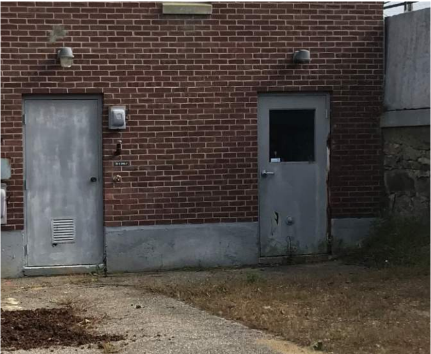
South Side Egress and Mech Room Entry
