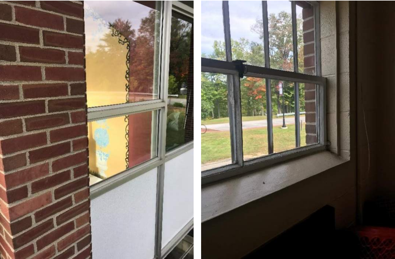
Typical Window (Exterior & Interior)
