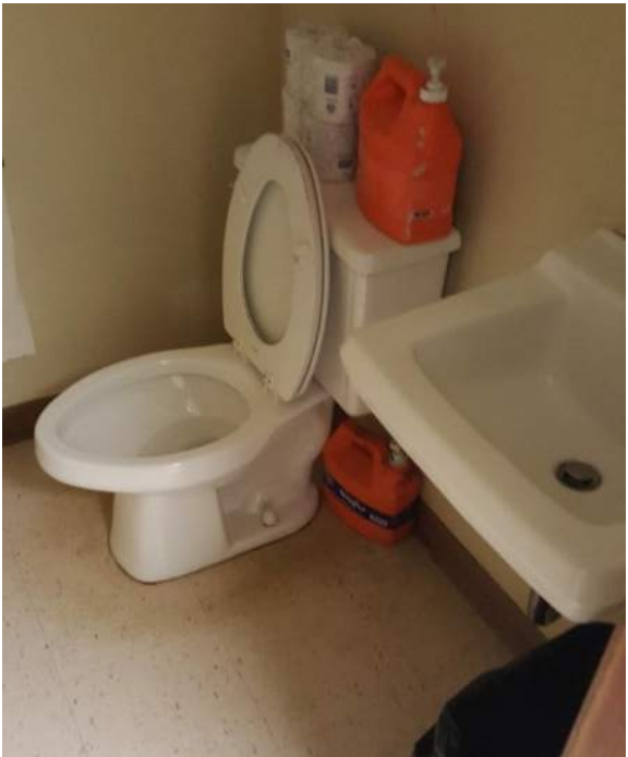
Public Bathroom Facilities
