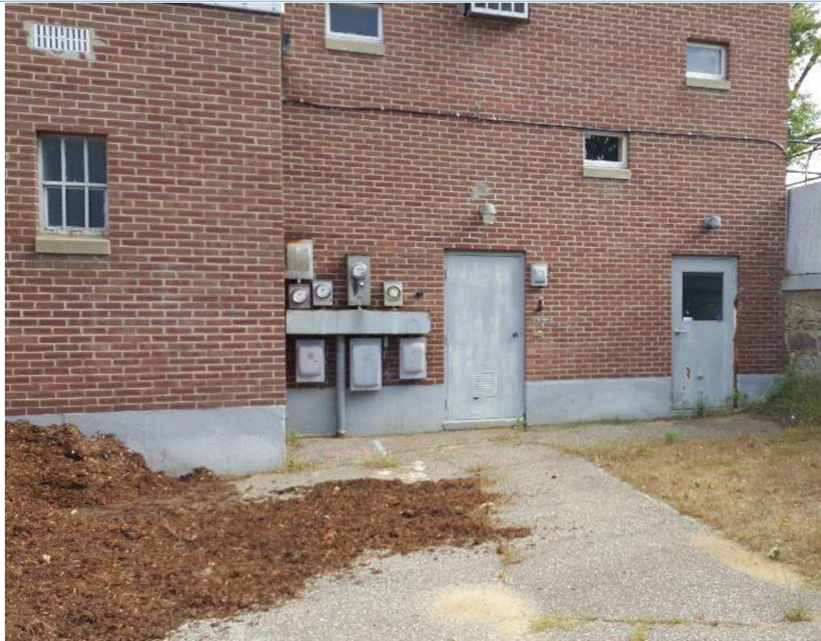
Abandoned Boiler Room and Location of Removed Oil Tank
