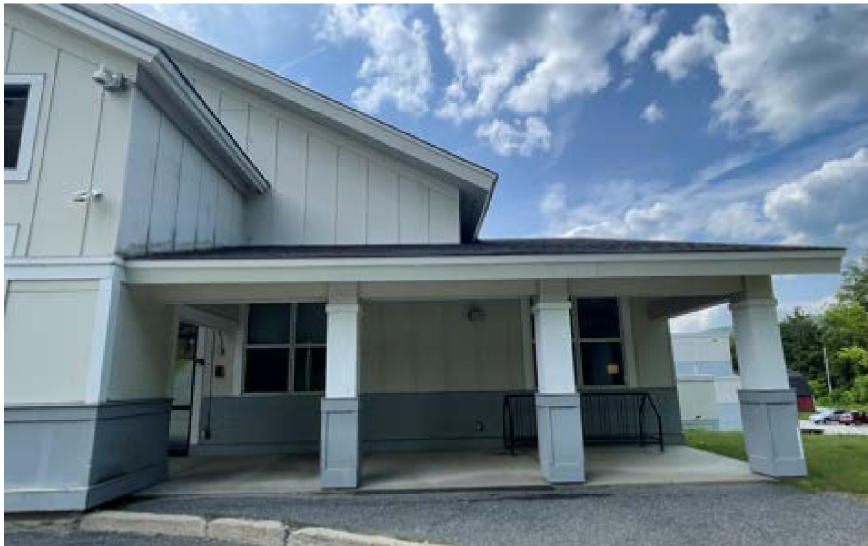
View of East Façade entry
