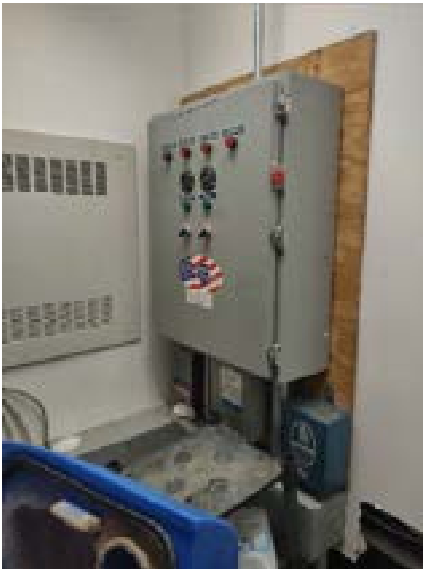
Control panel for well pumps.
