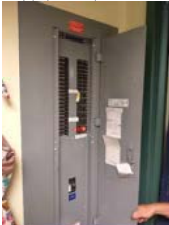
Fully populated panel with emergency fire circuit.
