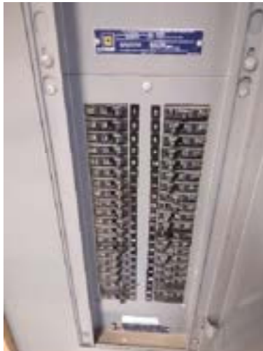
Fully populated panel with older breakers.
