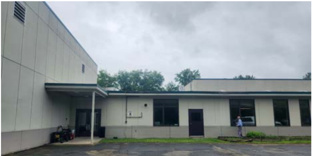
View of North East Corner towards gym
