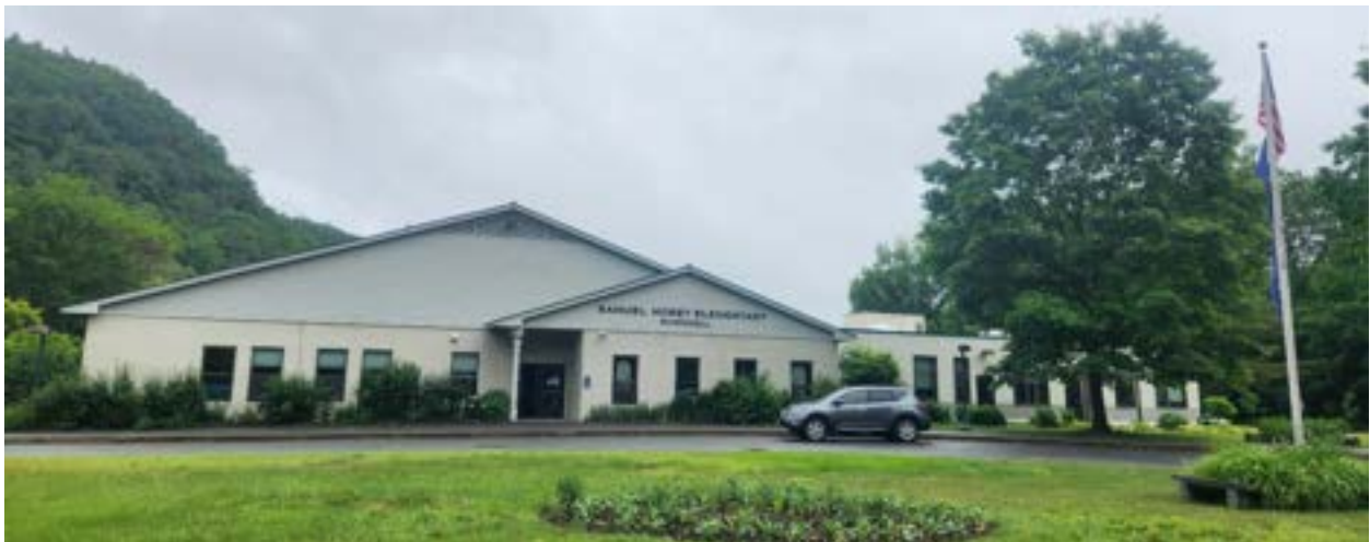
View of West entry Façade
