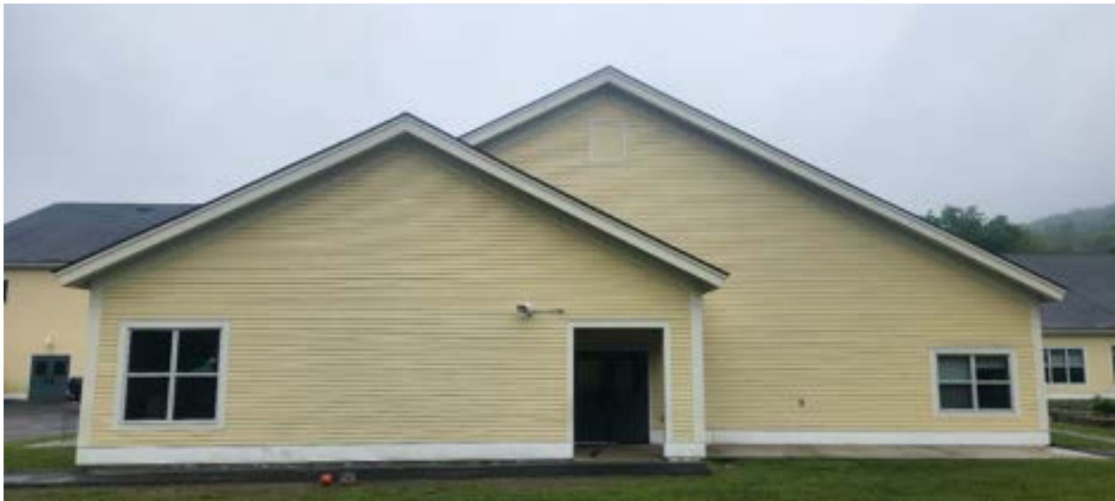
View of West Façade
