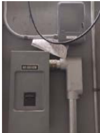
View of AHU room with electrical service panels for gym, HVAC, and FP.
