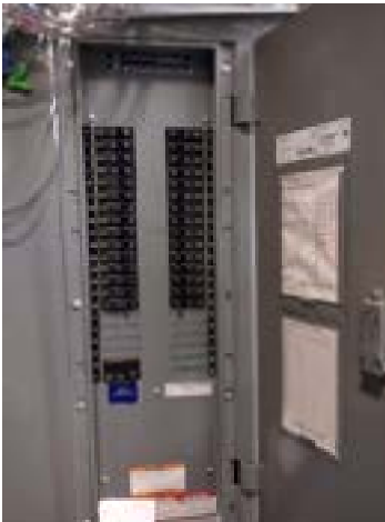
Fully populated panel with emergency fire circuit.
