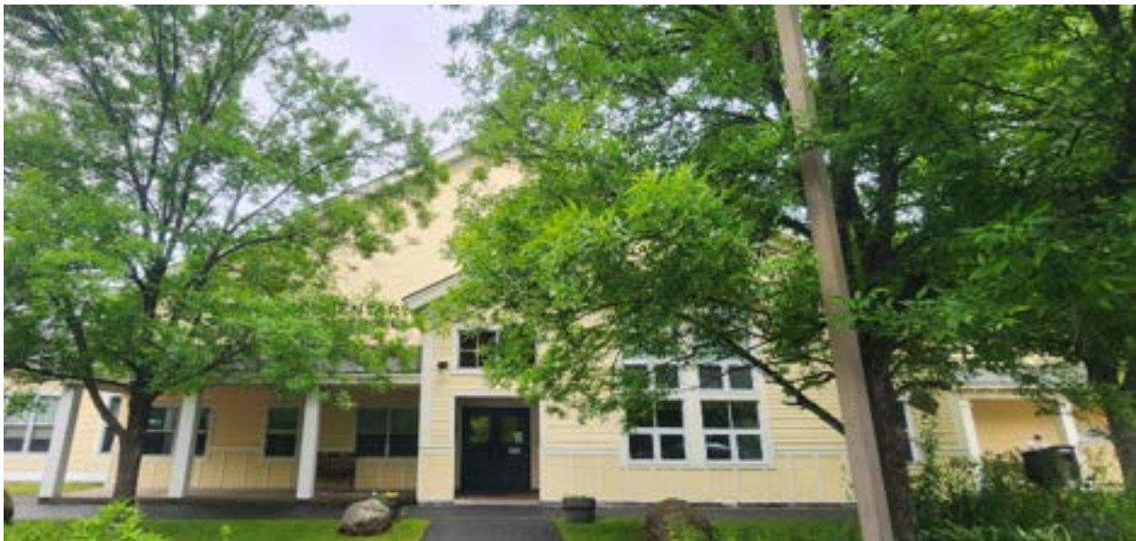
View of South Entry Façade
