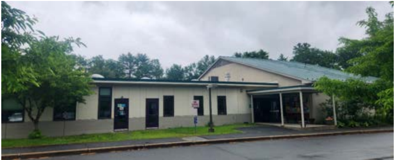
View of North Entry
