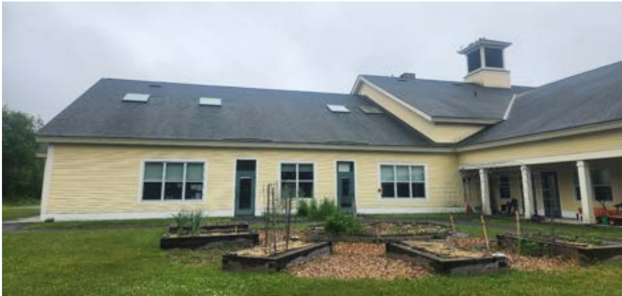
View of Northeast Courtyard looking East
