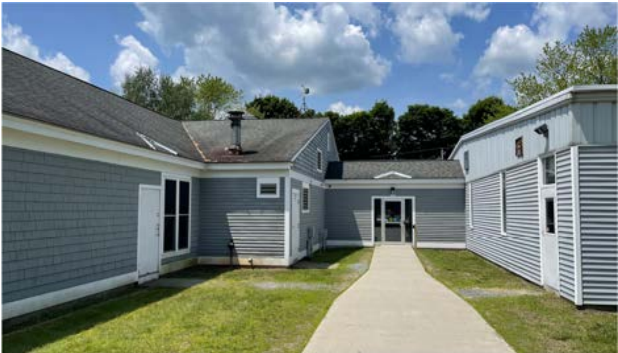
View of East Façade from Courtyard to Academy East Wing
