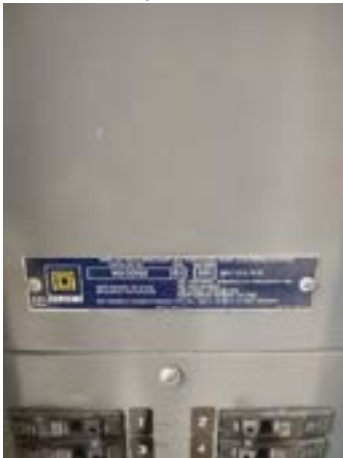
Older breakers in fully populated panel.
