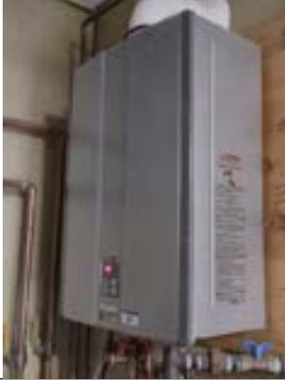
AHU Room boiler #3 – 15 years into a 30 year service life.
