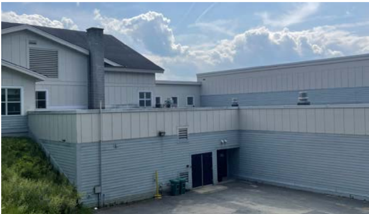
View of Northeast corner
