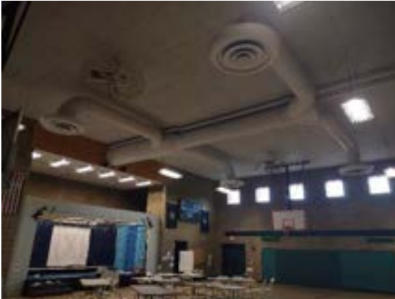
Ductwork diffuser arrangement in classroom – typical
