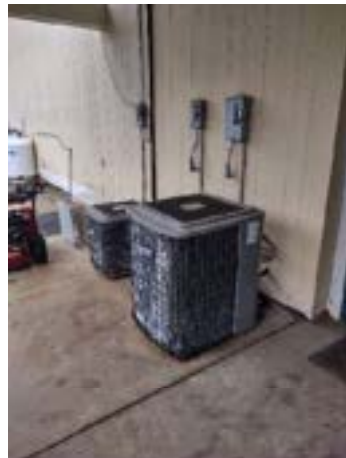
Split duct condenser unit.
