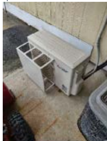
Split duct condenser unit.
