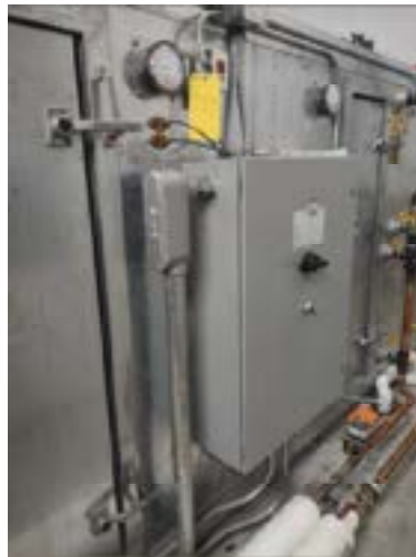
AHU controls in upper boiler room AHU space.
