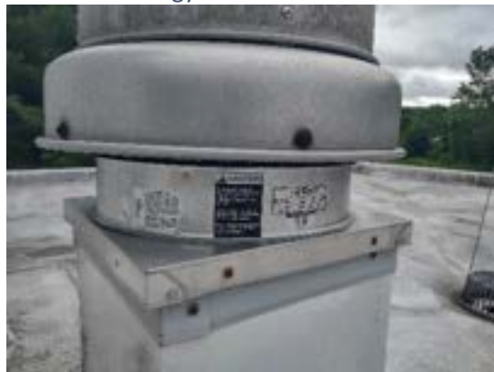
Exhaust fan on gym roof.
