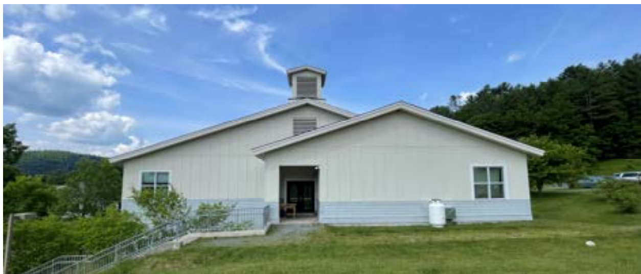
View of South Façade second floor
