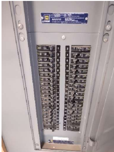
Fully populated panel with older breakers.
