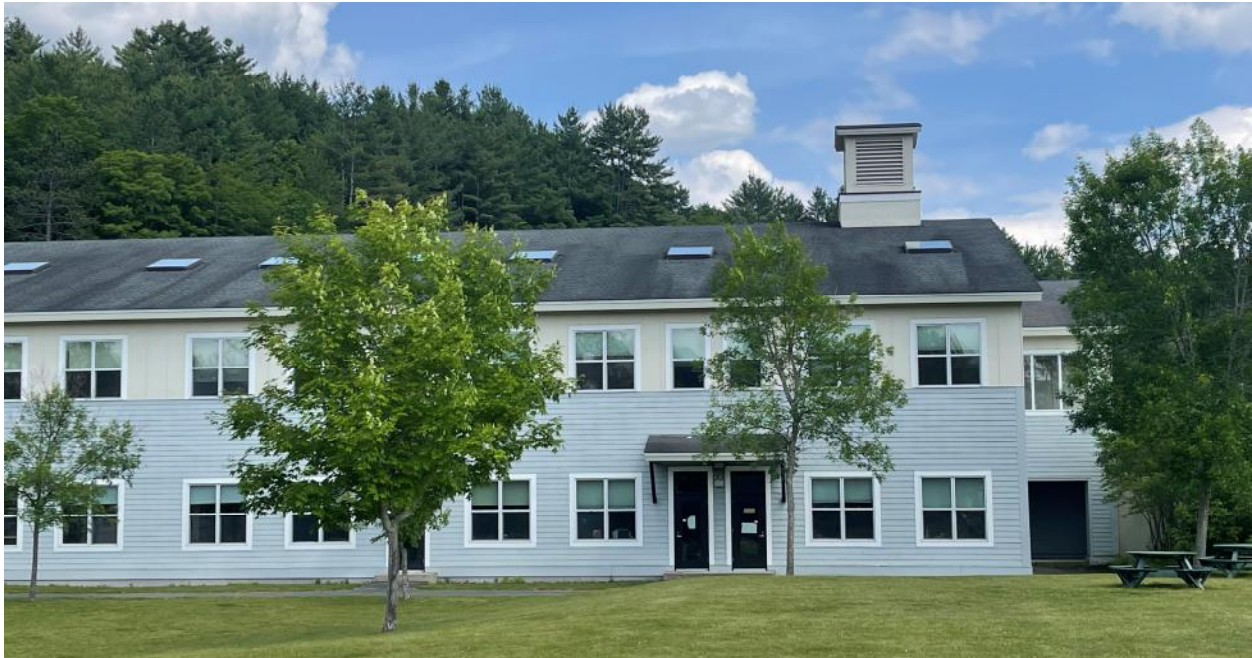
View of West Façade from courtyard
