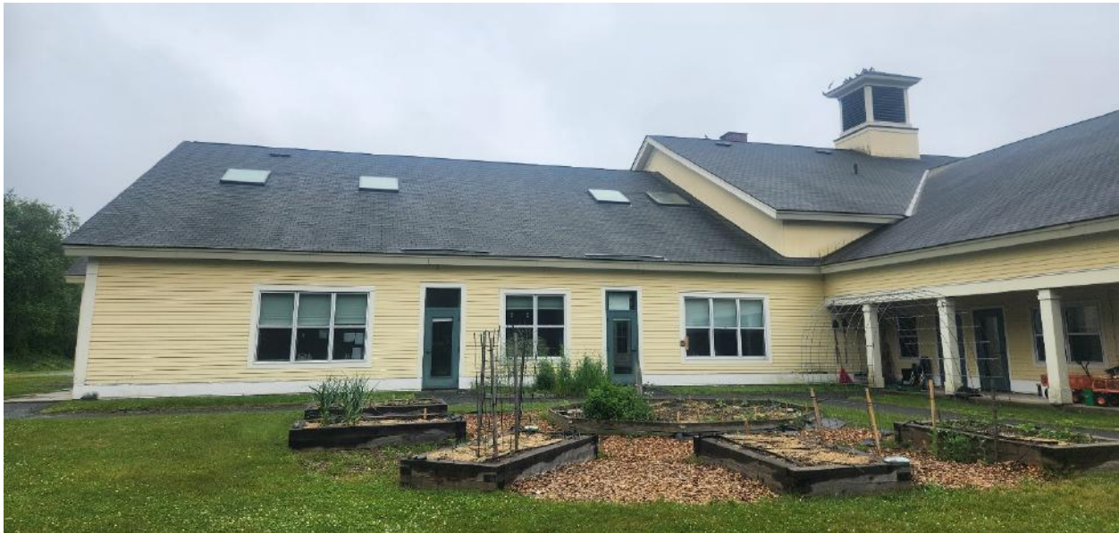
View of Northeast Courtyard looking East
