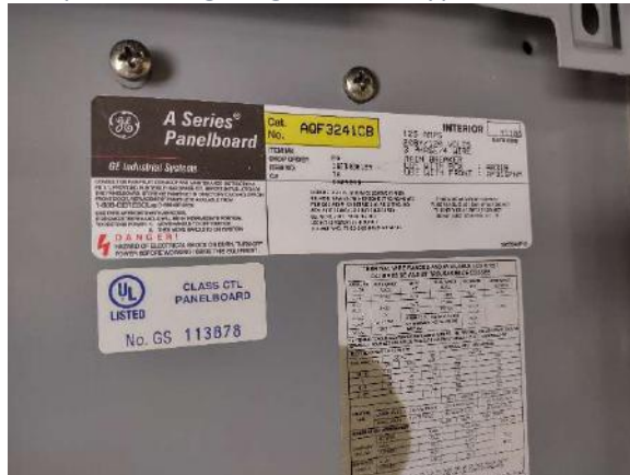
Sub panel for lighting circuits – typical
