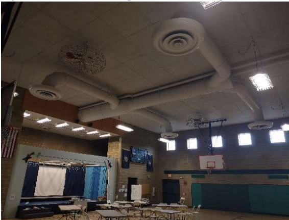
Ductwork diffuser arrangement in classroom – typical
