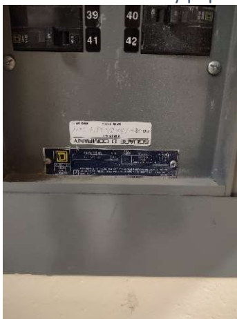
Older breakers in fully populated panel.
