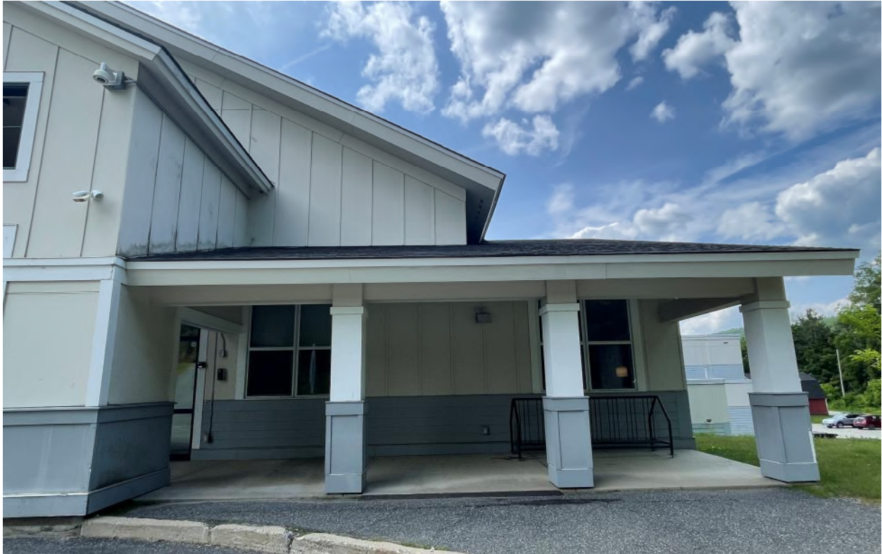
View of East Façade entry
