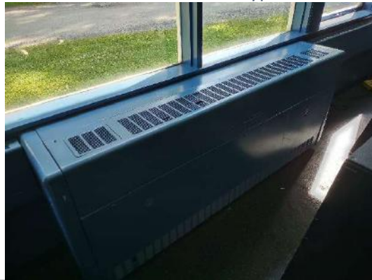
Unit heater and through wall AC in office area.
