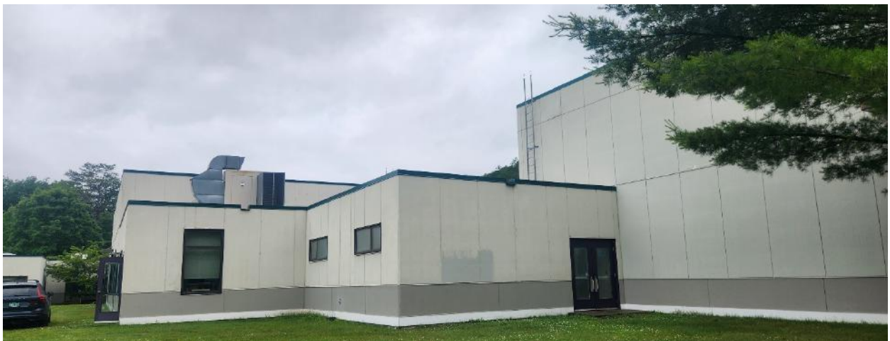
View of South East corner
