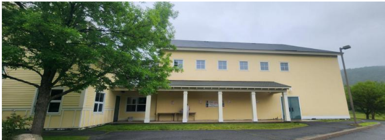
View of Southwest Corner
