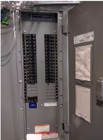
Fully populated panel with emergency fire circuit.
