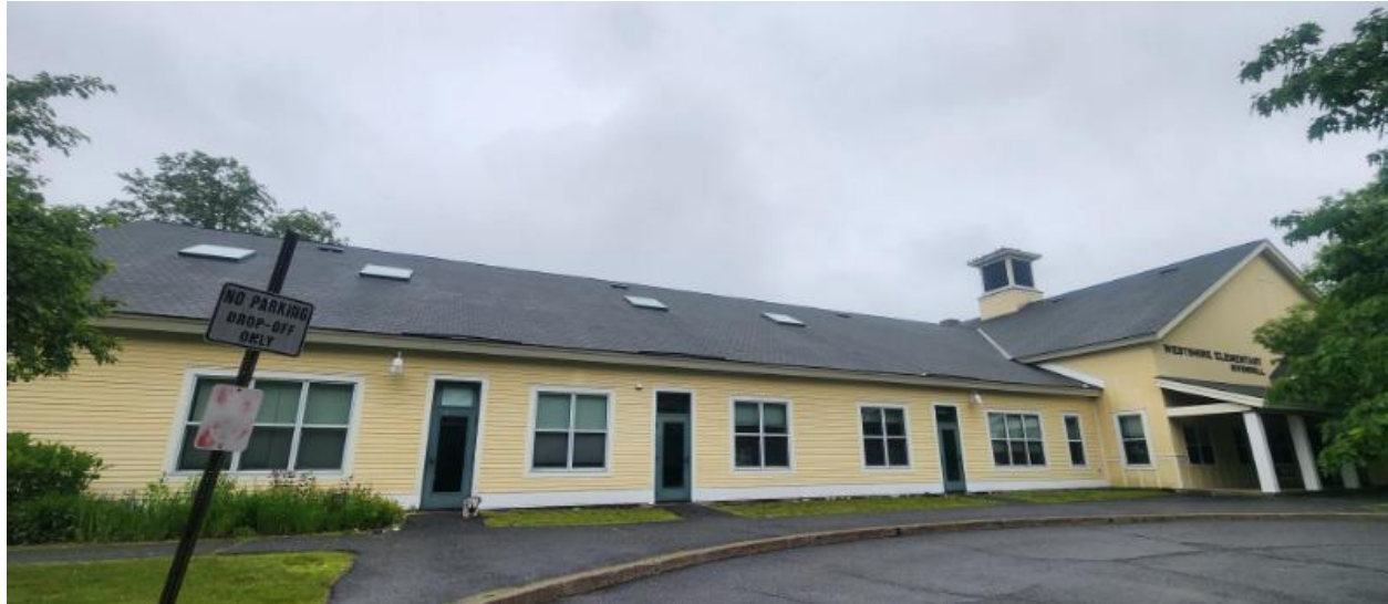
View of South Entry Façade
