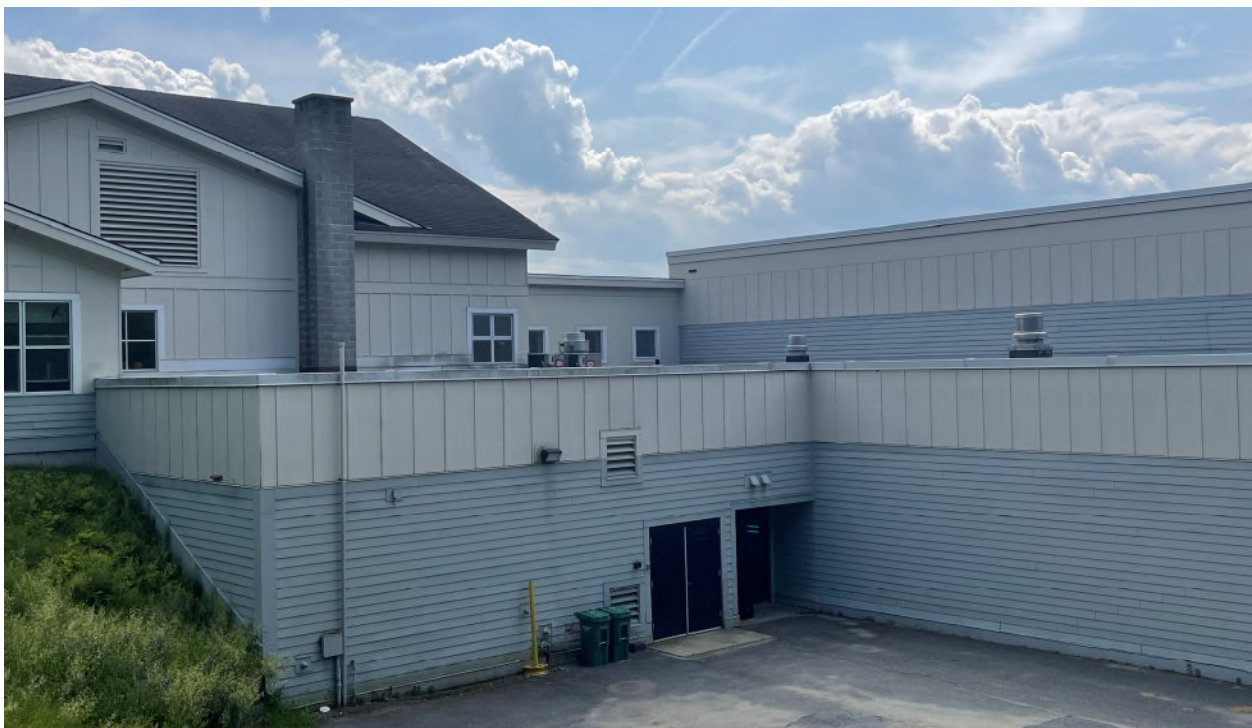
View of Northeast corner
