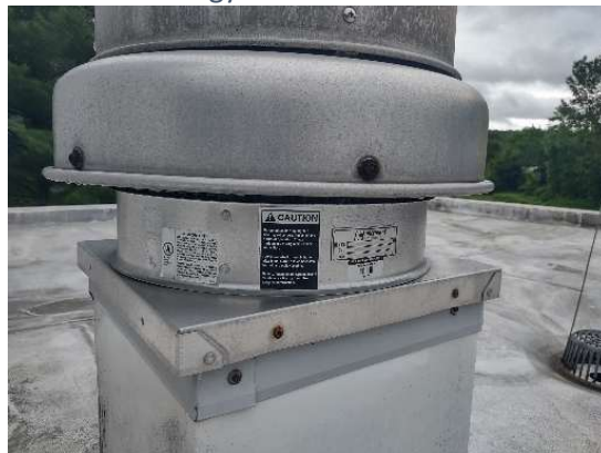
Exhaust fan on gym roof.
