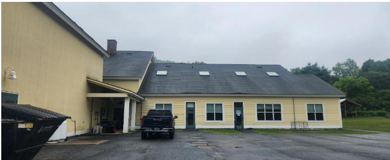
View of North Wing
