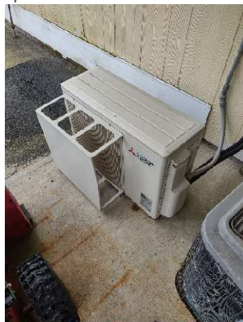
Split duct condenser unit.
