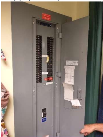
Fully populated panel with emergency fire circuit.
