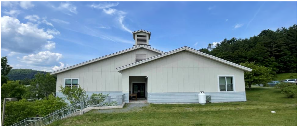
View of South Façade second floor
