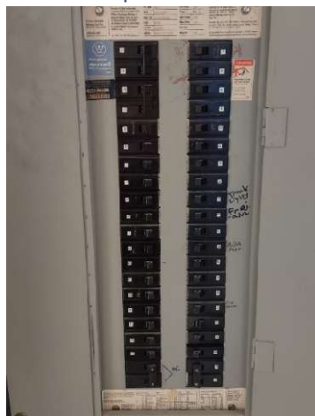
Functional panelboard shows signs of age.
