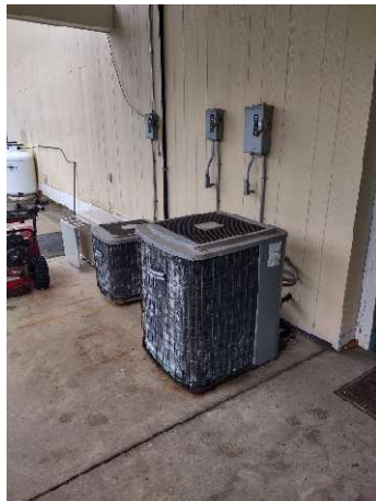
Split duct condenser unit.
