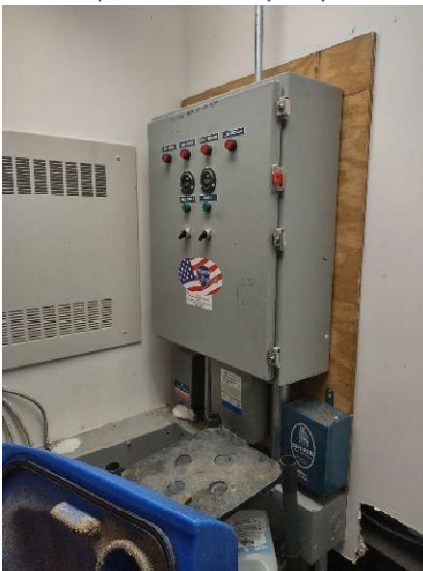
Control panel for well pumps.
