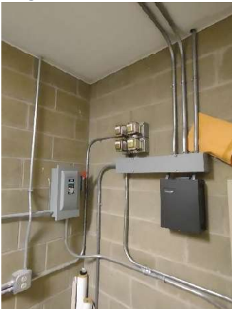
Stage AHU disconnect and wiring in conduit arrangement.
