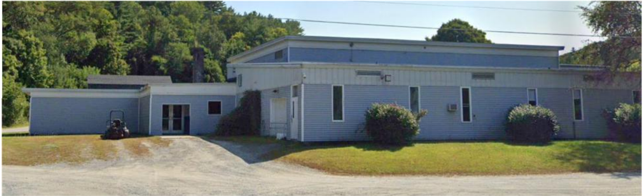
View of Northwestern Facade of Building
