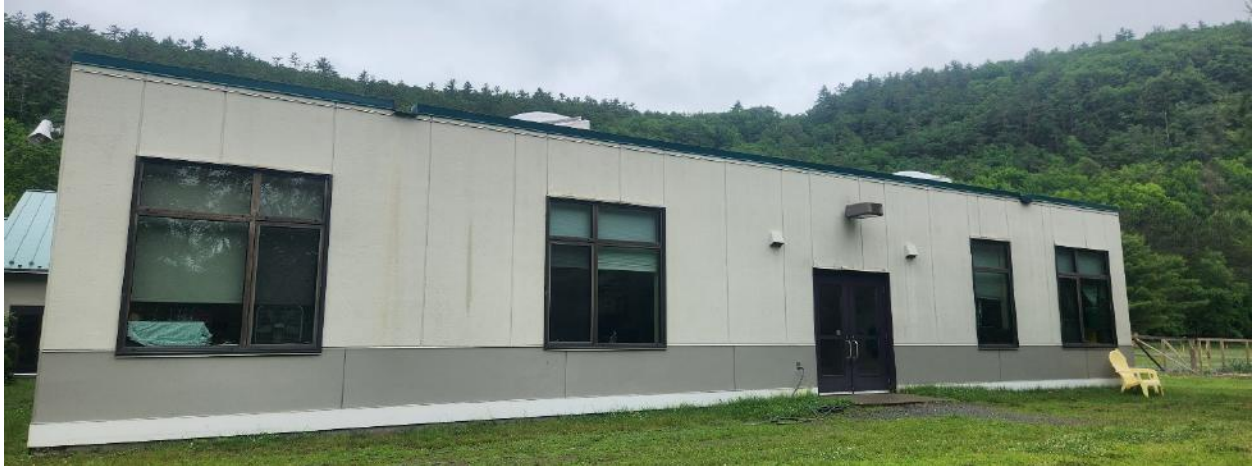
View of South Facade
