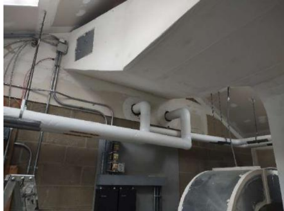
Control wiring for AHU arrangement.
