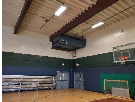
Terminal unit in classroom – typical.
