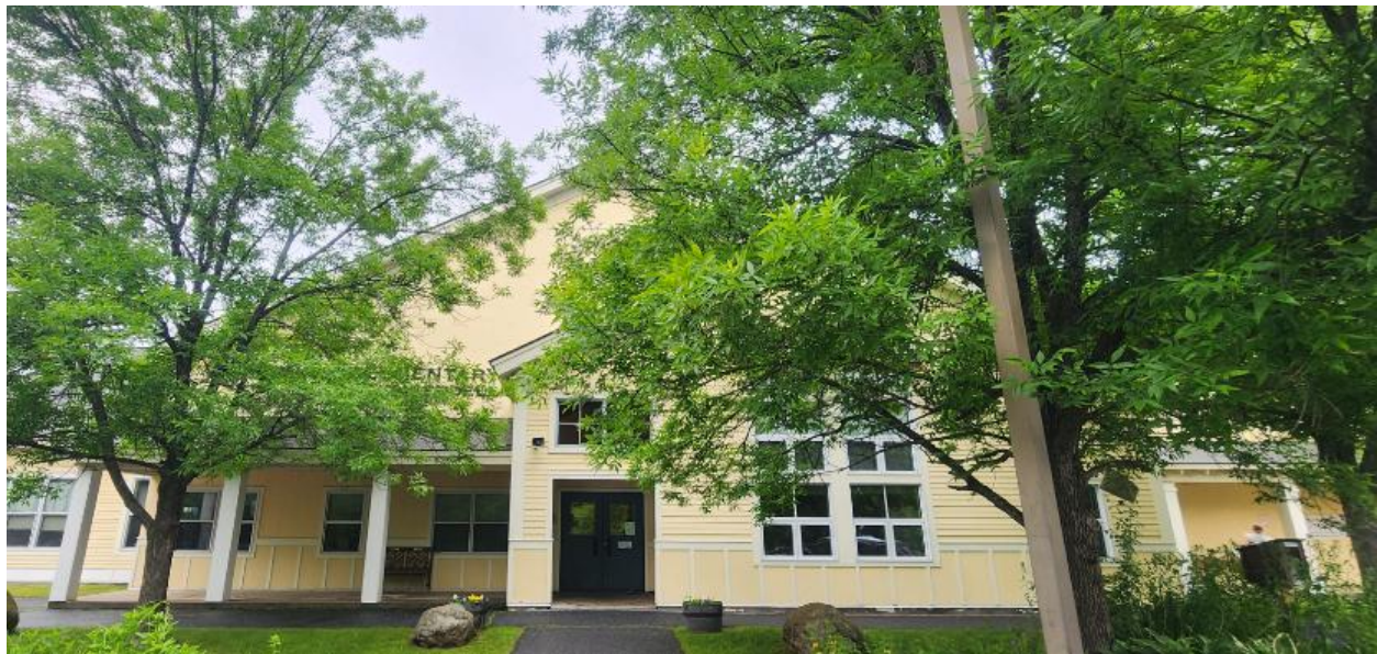
View of South Entry Façade
