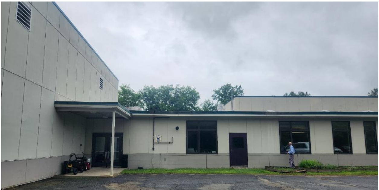
View of North East Corner towards gym
