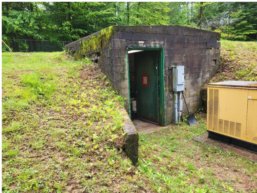
Photo 2 – Existing Well GPW 1 pump house. Taken 6/27/23
