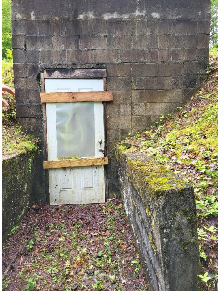
Photo 7 – Existing Well GPW 2 pump house. Taken 6/27/23
