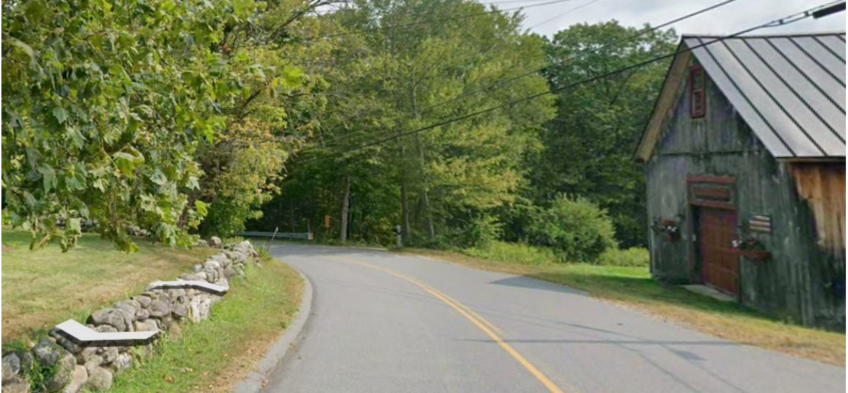
Figure 1. Horizontal curve limiting sight distance at 55 Christian Hill Road.
