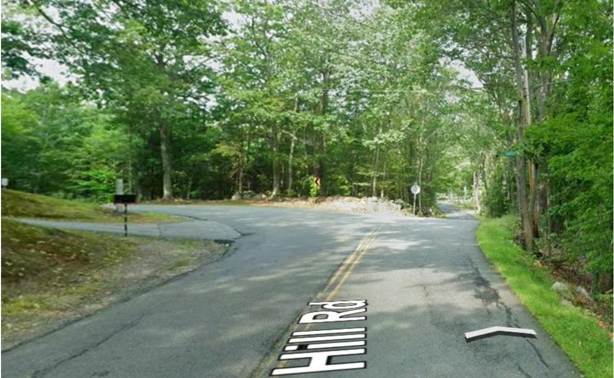
Figure 4. Horizontal curve limiting sight distance at the Christian Hill Road and Eaton Road intersection.
