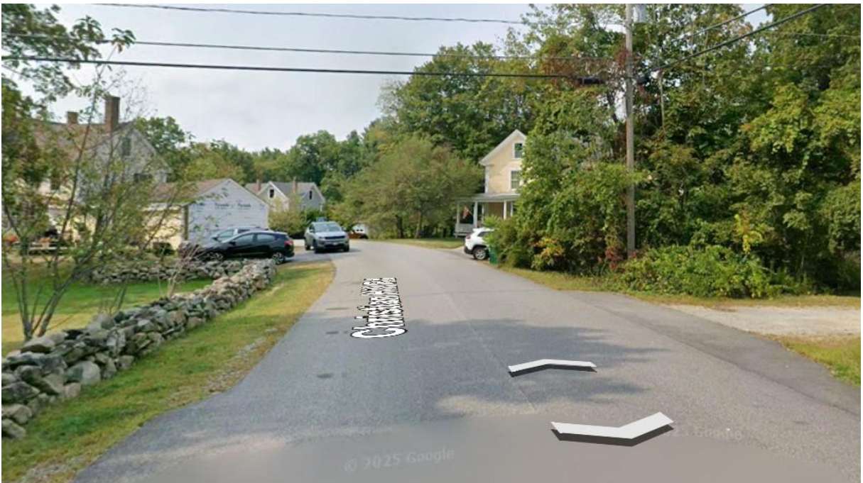
Figure 2. Horizontal curve limiting sight distance at 82 Christian Hill Road.
